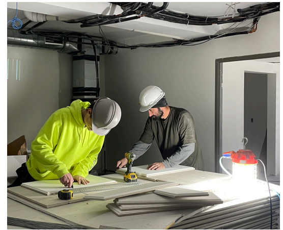
AT LEFT: The Heritage Center addition exterior is almost complete, as seen from 9th Street. ABOVE: Workers cut ceiling tiles to cover the conduits for heating, air conditioning, plumbing and electricity above them in the new addition.
